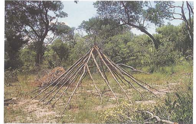
Terminalia sericea , resistant to wood-borers and light in weight, makes a suitable roofing structure
