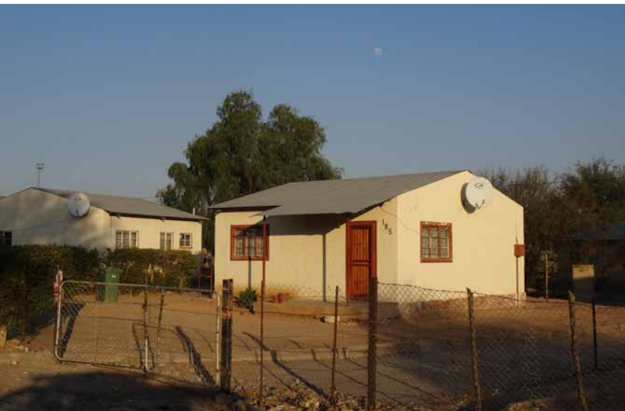
An old, low income house in Orvetoweni
