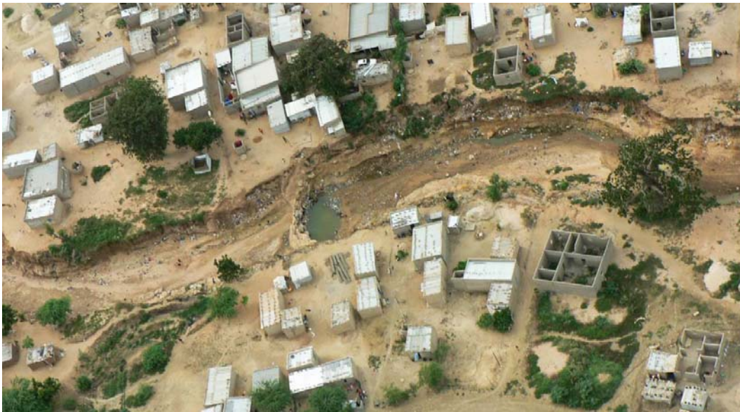
Blockages along drainage lines led to surges of water causing severe erosion which undermined the foundations of nearby homes.
