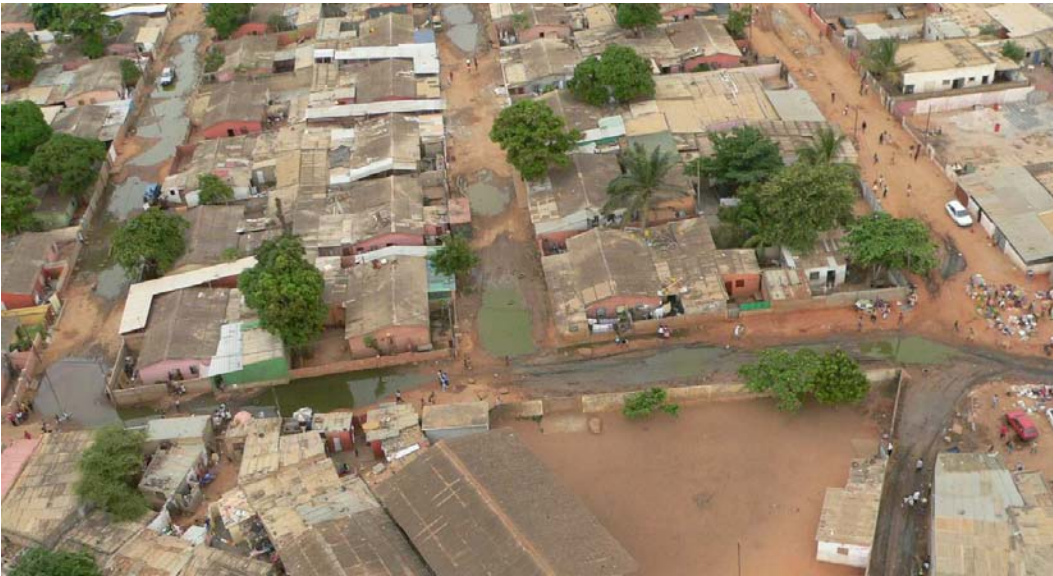
The remnants of sheet flooding as pools of water lying in roads. The houses around these roads would have been flooded after the heaviest rains.
